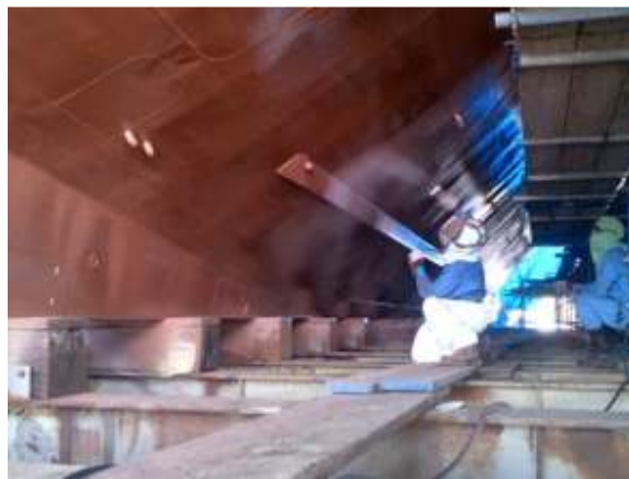
Picture 3 of spray angle and distance minimizing over spray
